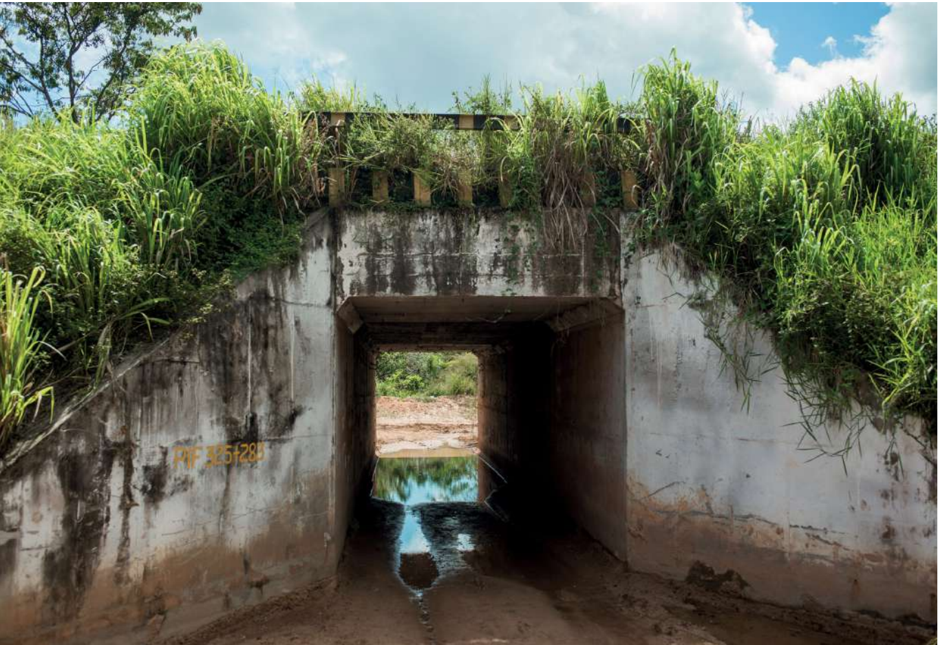
Underpass access to the communities, built by Vale. June 2021.
